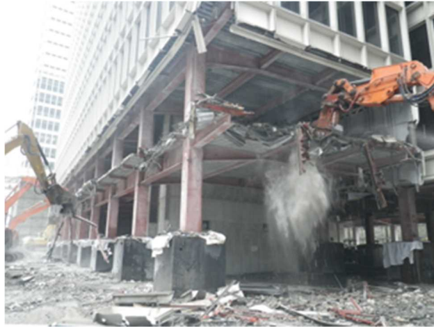
(a) The removal of the floating dust in building site
