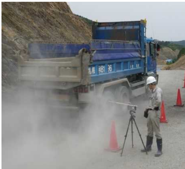
(b) The removal of the floating dust in civil construction
