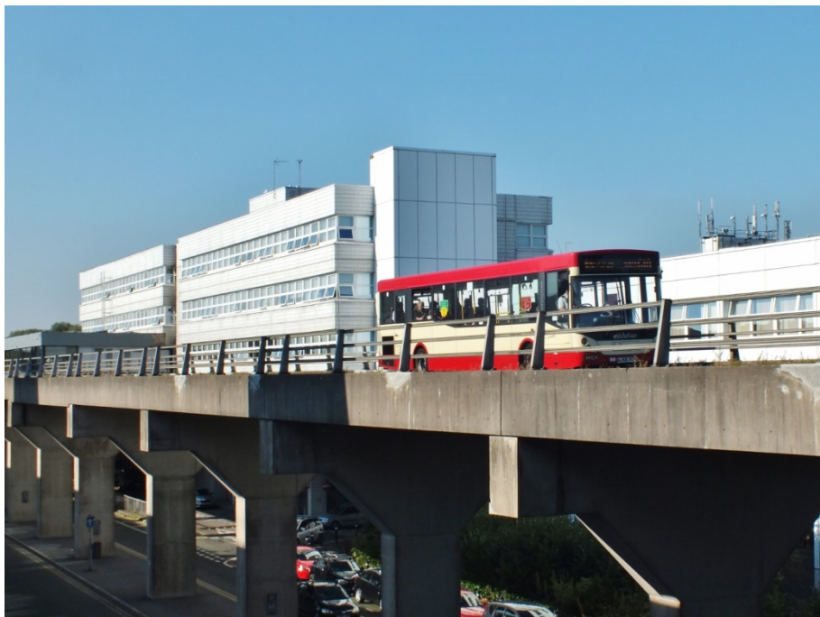
Figure 2.1: Elevated Section of Runcorn Busway
