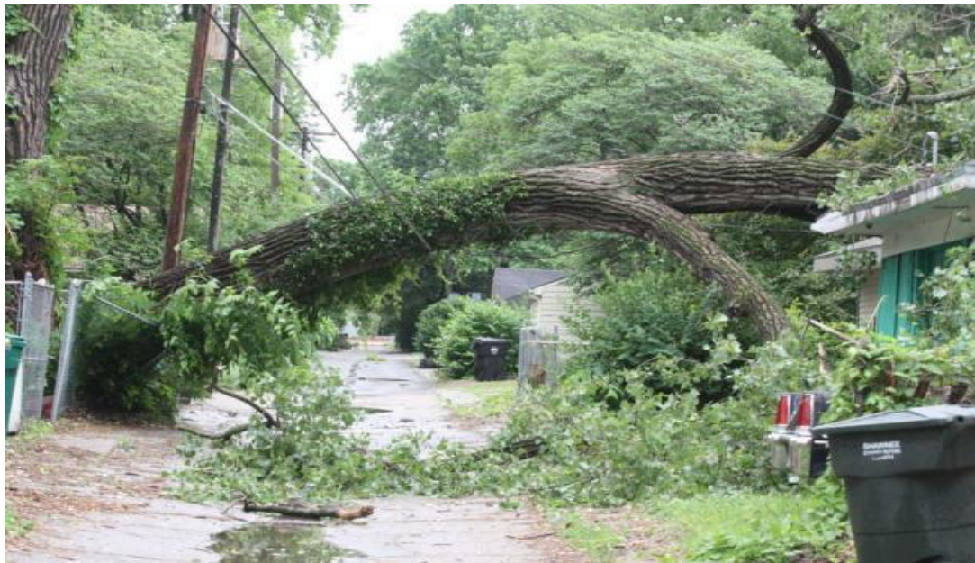
Figure 1-2 Distribution line interrupted by fallen tree
