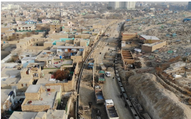
Fig. 2 Aerial photo of the study area during development.
