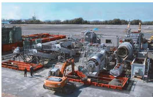
Fig. 11 Cleanup of contaminated soils by washing equipment 5) .
