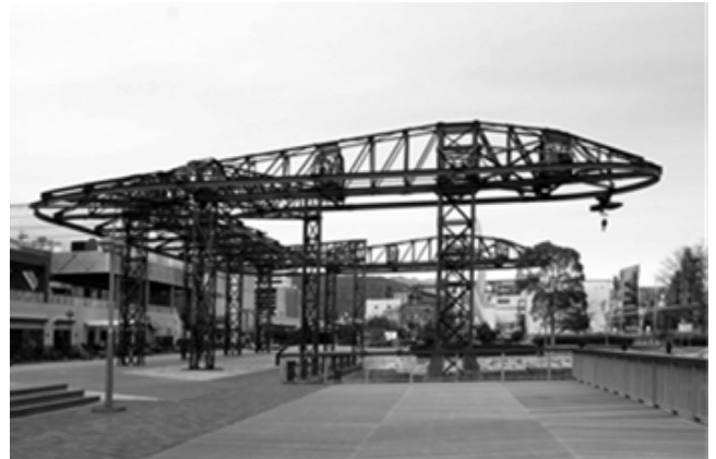
Fig 4. Present telpher of the Port of Shimizu
