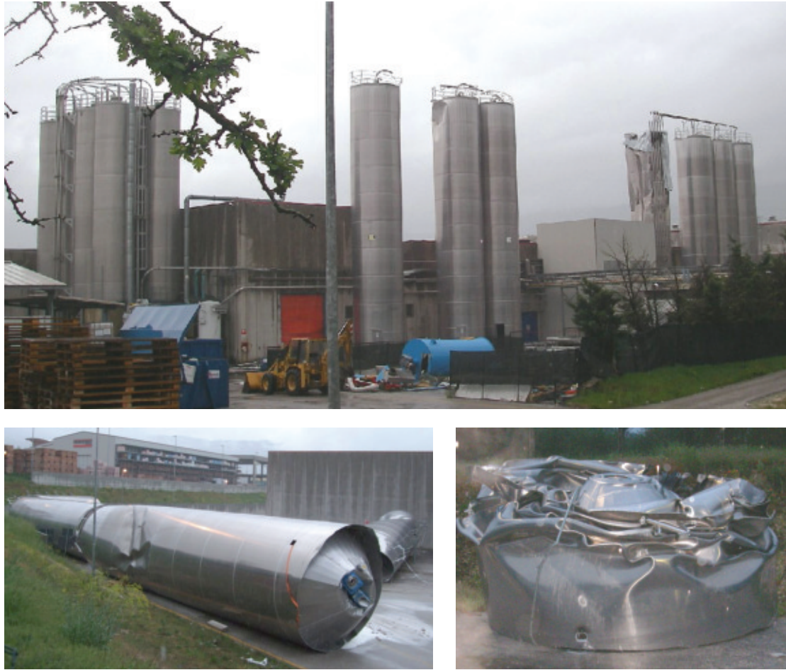
Figure 42. Views of buckled silos.
