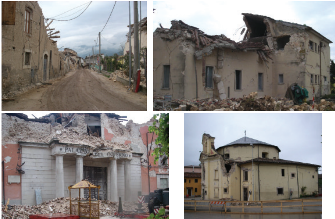
Figure 35. Examples of masonry building damage.
