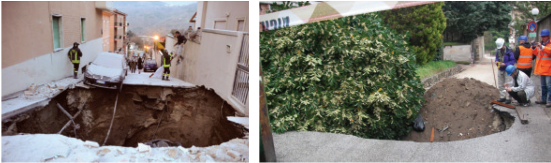
Figure 29. Sinkholes in L'Aquila.
