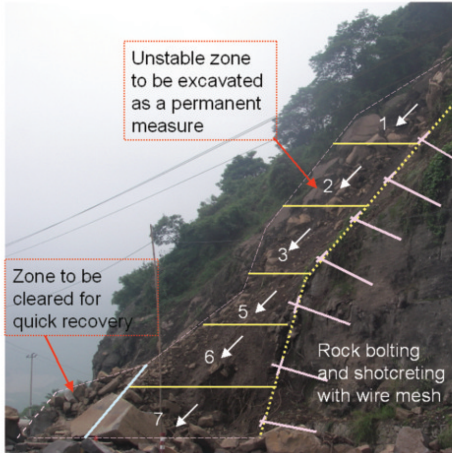
Figure 14. Proposed quick recovery and permanent measures for the restoration of failed slopes (Hamada and Aydan, 2008)
