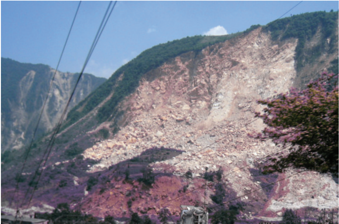
Figure 8. A view of the Xuankou (Yingxiu) landslide
