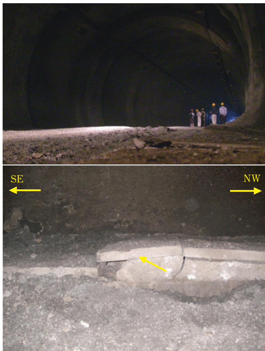
Figure 22. Views of repaired damaged section of the tunnel near the Zipingpu dam
