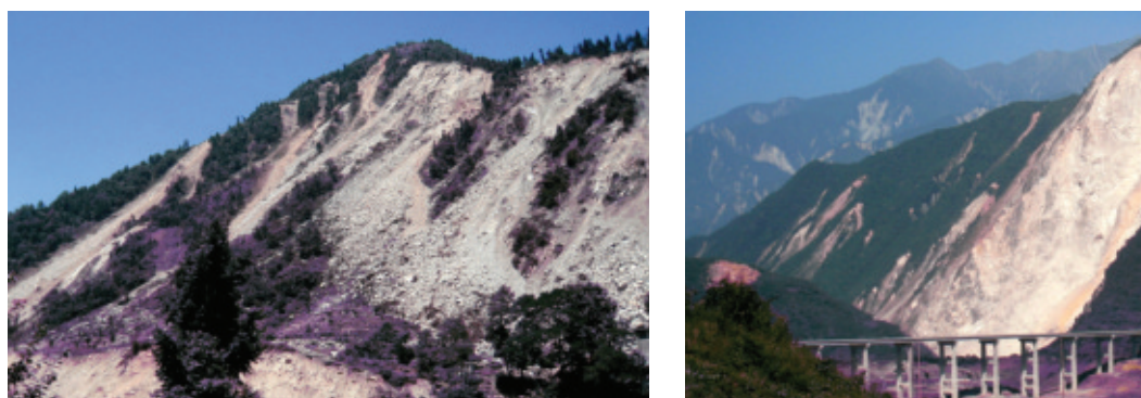
Figure 6. Spectacular surficial rock slope failures
