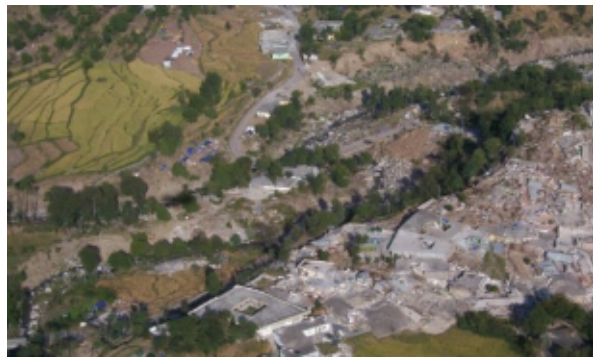
(b) Slope failure in Balakot
