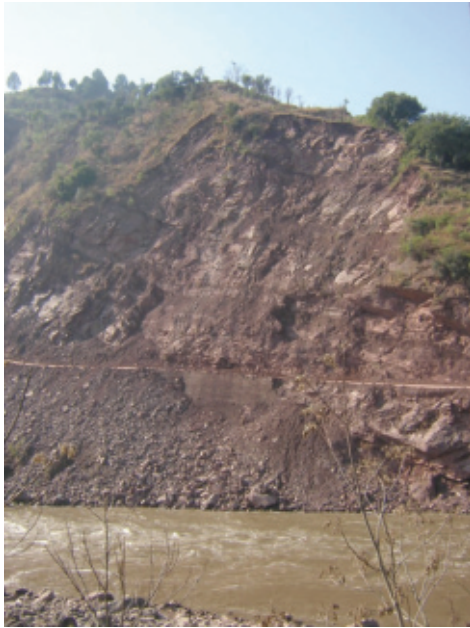
(a) Flexural toppling failure
