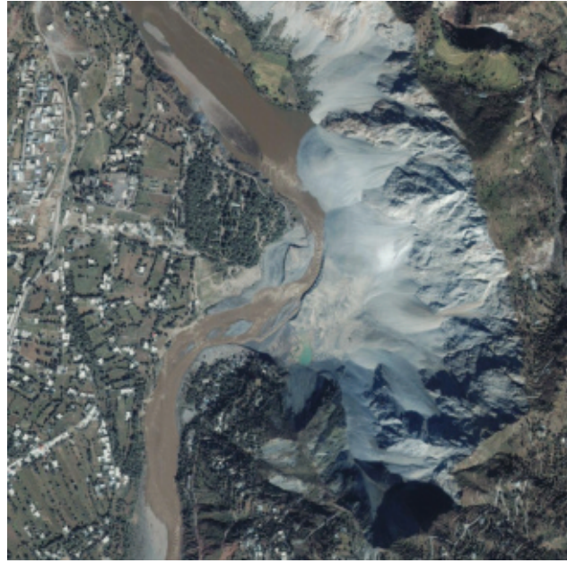
(b) Surficial failure of fractured dolomite
