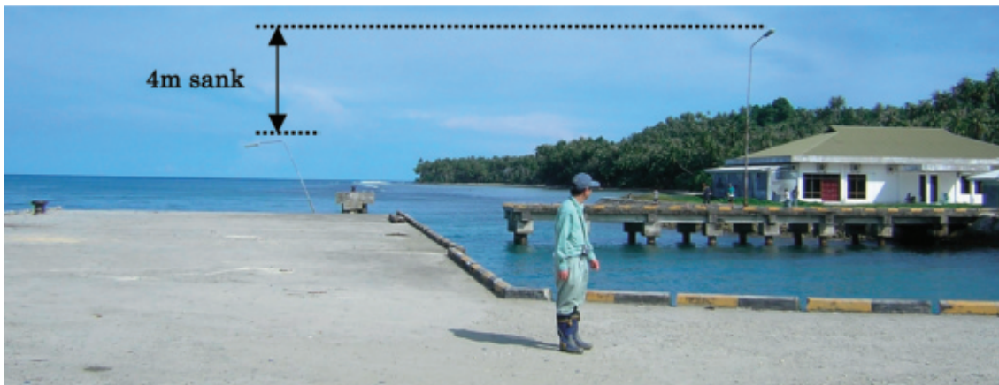
(b) Sank part of the wharf at Telukdalam new port
