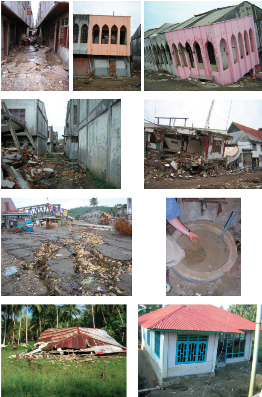
Figure 9 Effects of liquefaction and lateral spreading on RC buildings
