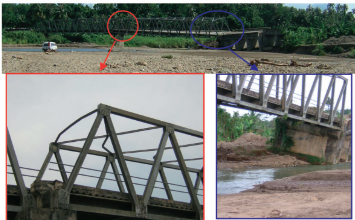
Figure 15 Gawo Bridge nearby Tetelesi
