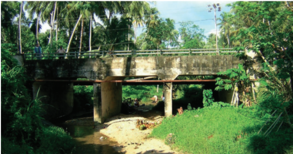
Figure 18 Non-damaged RC box culvert
