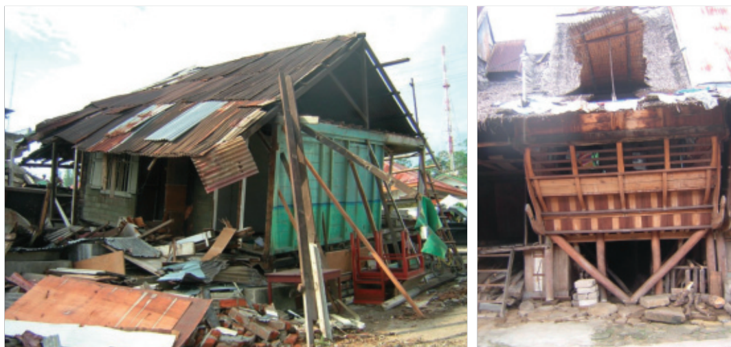
Figure 12 Damage to wooden houses and schools
