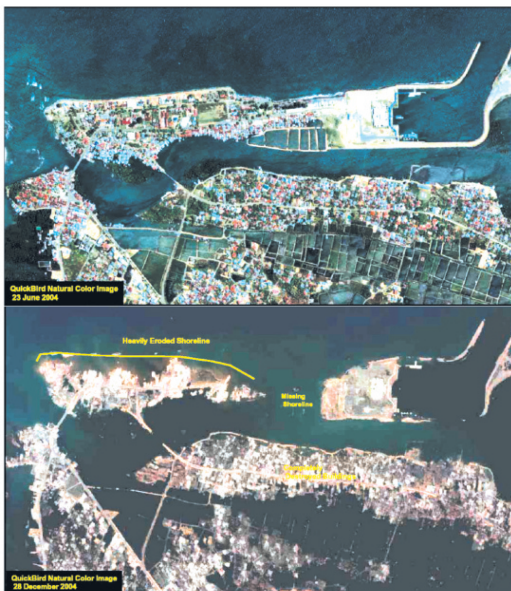
Figure 11 Satellite views of Banda Aceh port before and after the earthquake
