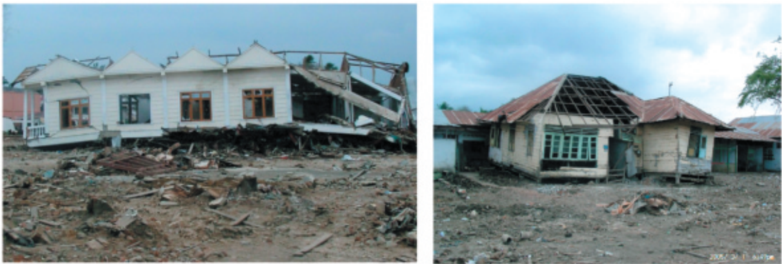
Figure 16 Damage to wooden houses
