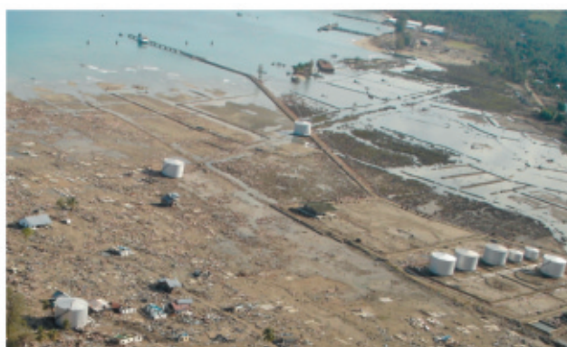
(b) Damaged oil tank farm and displaced tanks
