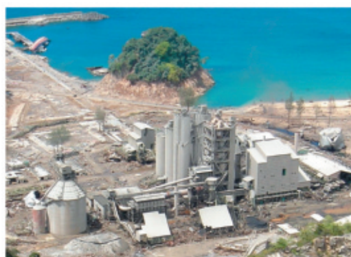
(a) Damaged cement factory
